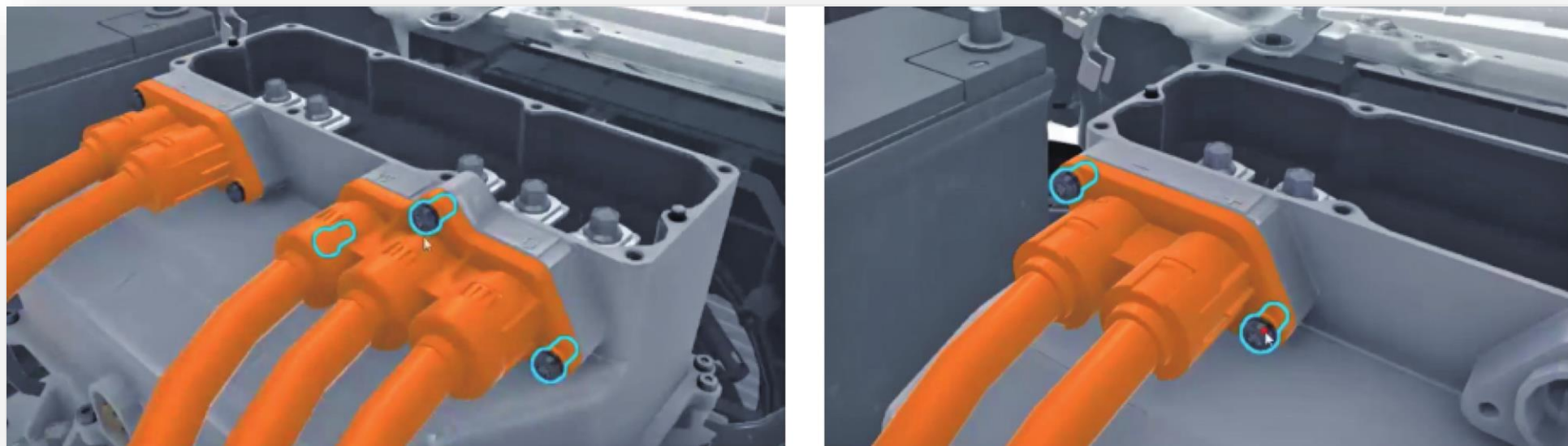
拆卸插接器固定螺栓
